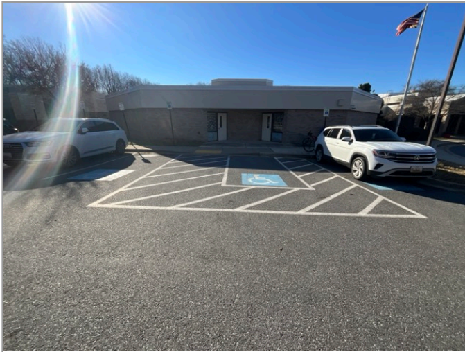
OVERVIEW OF ACCESSIBLE PARKING AREA
