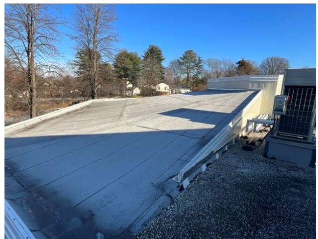
6 - SECONDARY ROOF OVERVIEW
