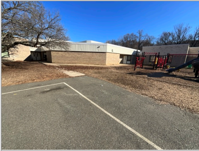
ACCESSIBLE ROUTE TO PLAYGROUND
