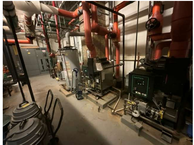
22 - OLD BOILER ROOM
