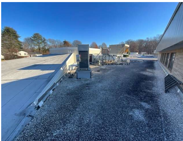
5 - PRIMARY ROOF OVERVIEW
